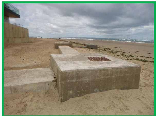
Outfall structure has been re-constructed and is in as-built condition (/C0602C05)
