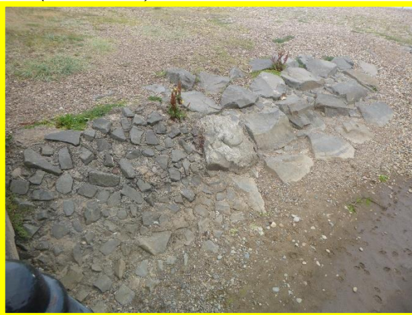
Grouted rock revetment to north of beck in fair condition (/C0704C06)
