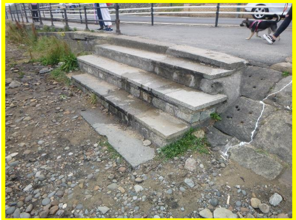
Repairs to steps in fair condition (/C0704C06)
