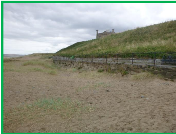
Well vegetated slope above masonry wall CBU E52/7
