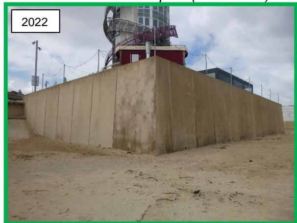
Concrete sea wall at Redcar Beacon note beach levels obscure concrete apron (/C0602C03)
