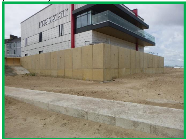
New Regent Cinema seawall (/C0602C05)
