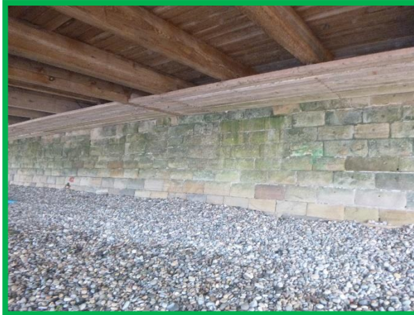
Masonry wall beneath Saltburn Pier (/C0702C04)
