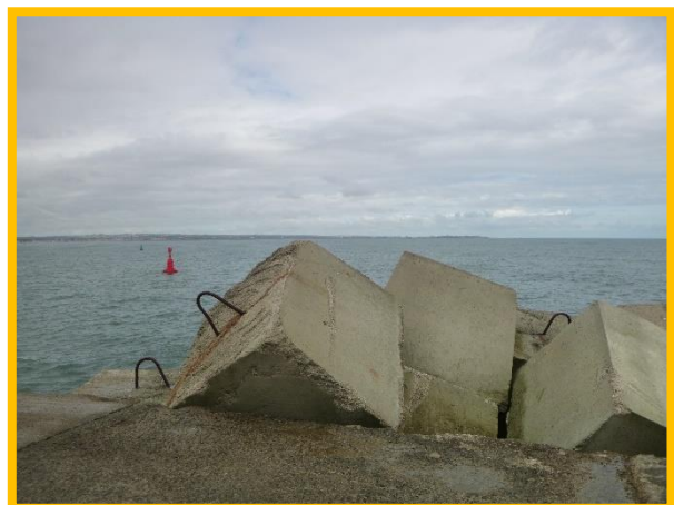
Recently placed concrete blocks at seaward end of structure (/C0506C01)
