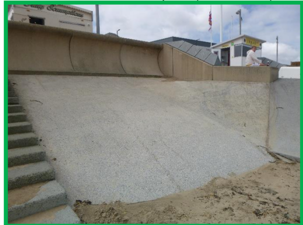
In-situ cast concrete transitions in good condition (/C0602C03)
