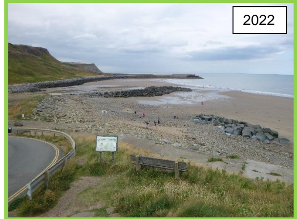
Modified defences to the east of Kilton Beck, 2022. Note: detached breakwater
