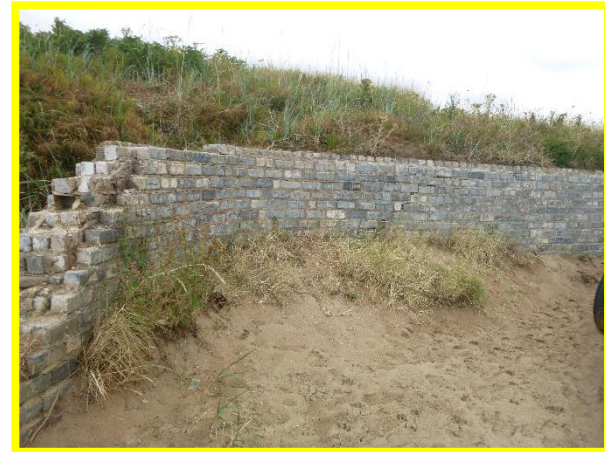
Masonry wall south east of beach entrance (/C0702C01)
