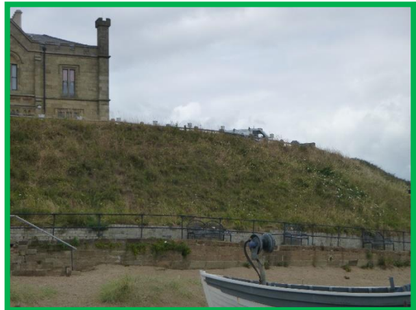
Well vegetated slope above masonry wall CBU E52/7
