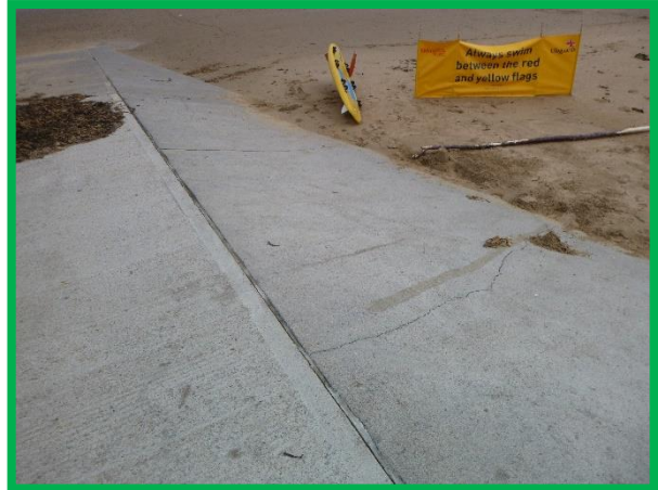
Joint sealant on slipway in fair condition (/C0602C03)
