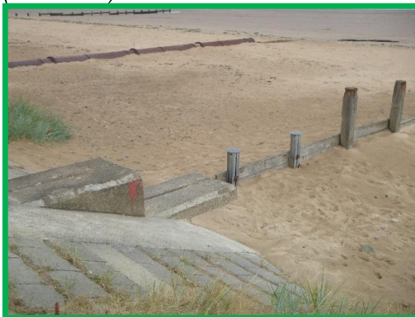
Recently repaired groyne along The Stray (/C0603C01)
