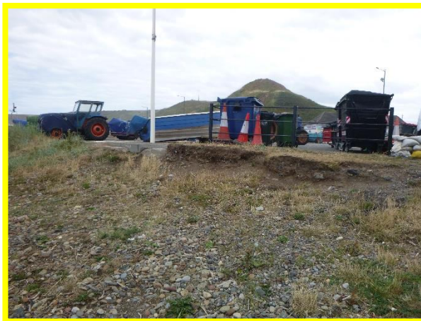
Vegetation establishment fronting car park (C0704C02)
