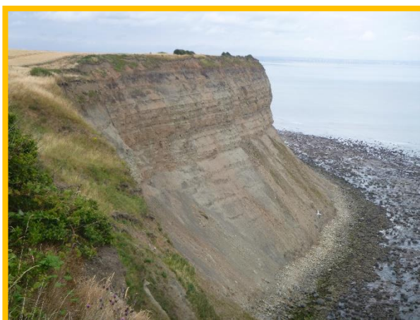
E54/4 looking northwest along Hunt Cliff showing active cliff face and debris apron (Partly Active)
