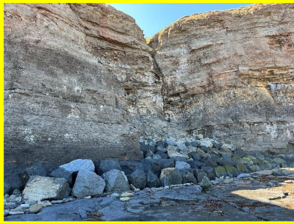
E59/1 Rock armour located at toe of cliff to the west of Cowbar Cottages
