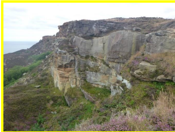
E58/5 Upper looking towards Rock Cliff. Locally Active upper sections and Partly Active lower sections.
