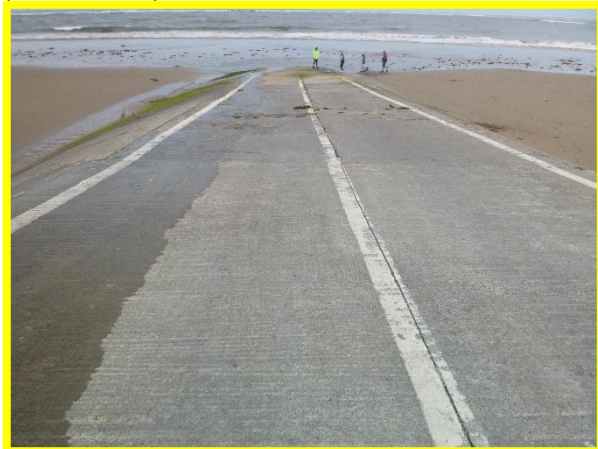
Slipway in fair condition (/C0602C02)
