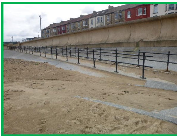
Slipway in very good condition (/C0602C04)
