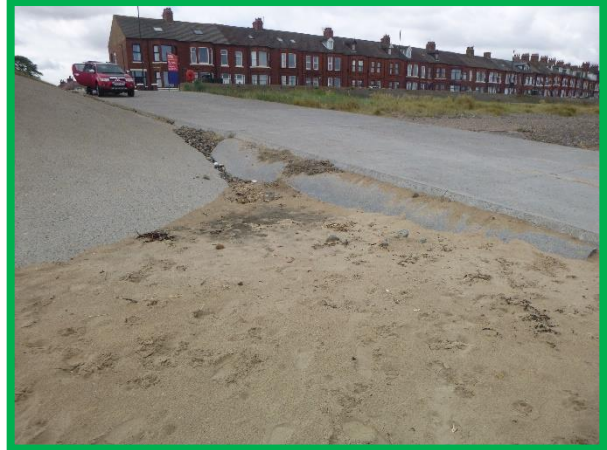
Concrete slipway in good condition (/C0602C01)
