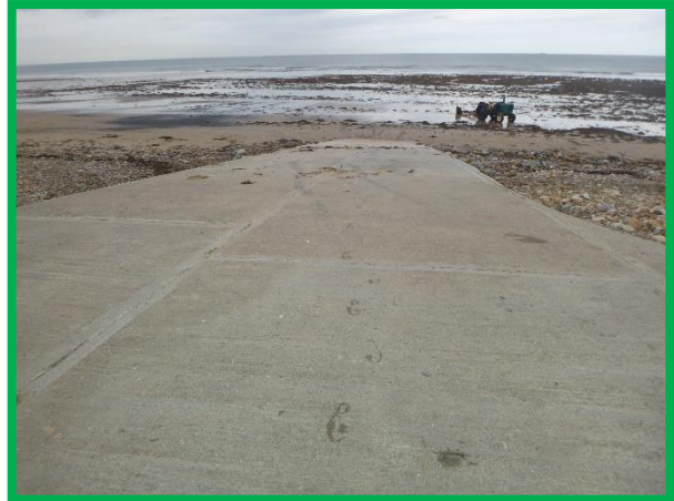
Concrete slipway adjacent Ship Inn car park (/C0704C03)
