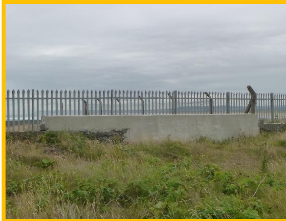
Repairs to wall on breakwater crest (/C0506C01)
