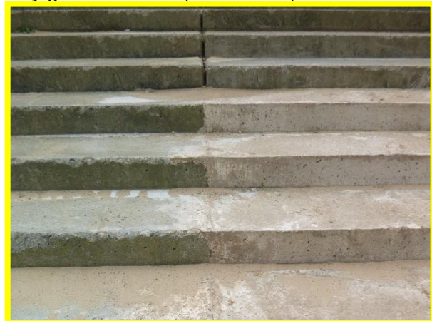
Close up of repair (/C0602C03)
