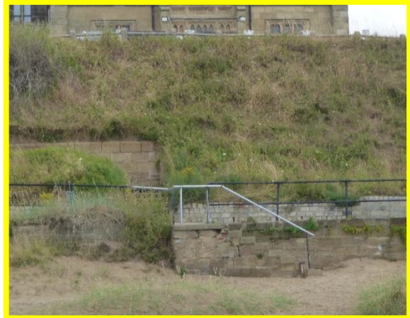
Steps in fair condition new handrail fitted since 2020 (/C0702C03)
