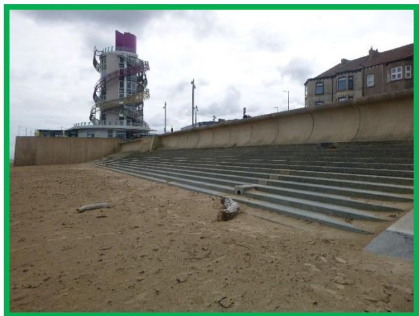
Stepped concrete revetment with recurve wall in very good condition (/C0602C03)
