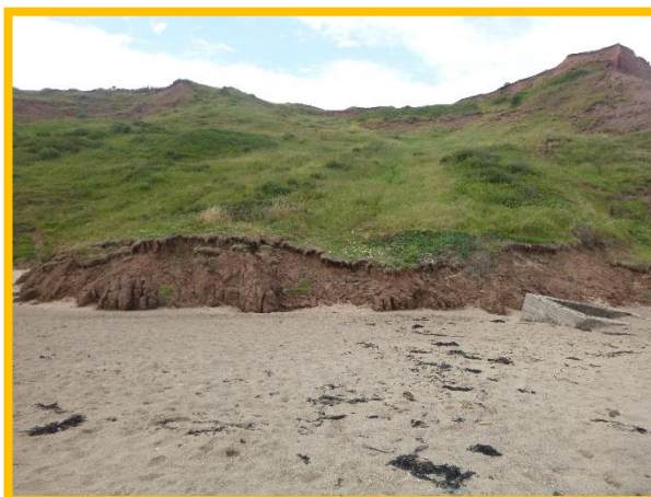
Evidence of past mudslides and erosion along the toe of E55/1 .
