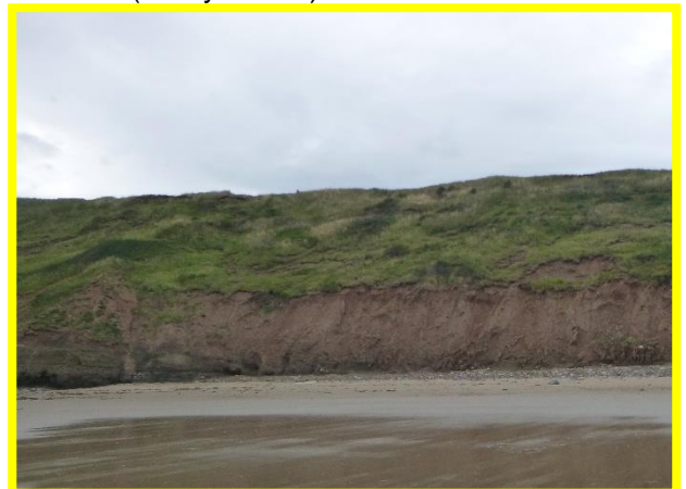
E53/5 ongoing erosion of the toe directly east of Saltburn (Locally Active).
