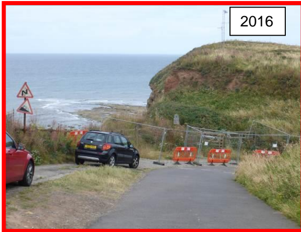
E60/1 Closure of access to Cowbar Nab in 2016, in 2018 the access appeared in very similar state with the same Heras fencing and plastic barriers still in use.
