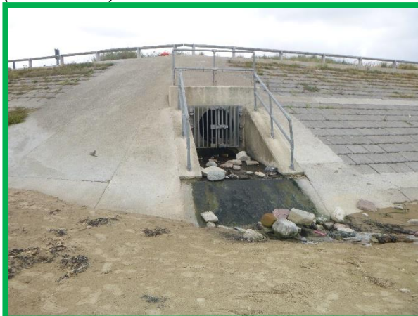
Outfall at south eastern end of (/C0603C01)
