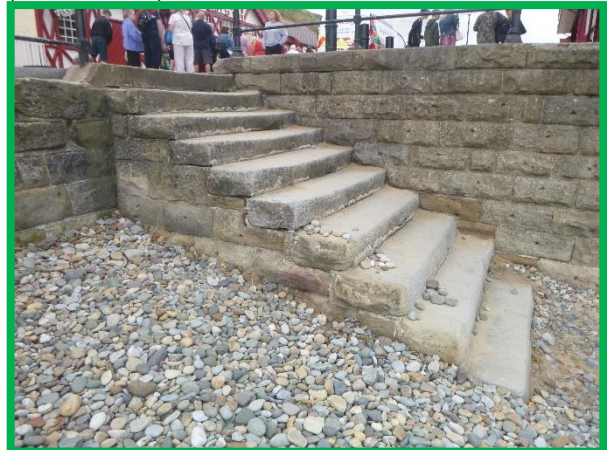
Beach access steps south of Saltburn Pier (/C0702C04).
