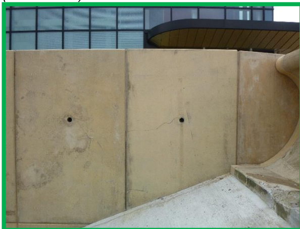
Pre cast concrete wall (/C0602C05)
