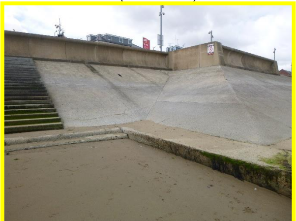
Concrete apron of slipway in good condition, despite being exposed.(/C0602C01).
