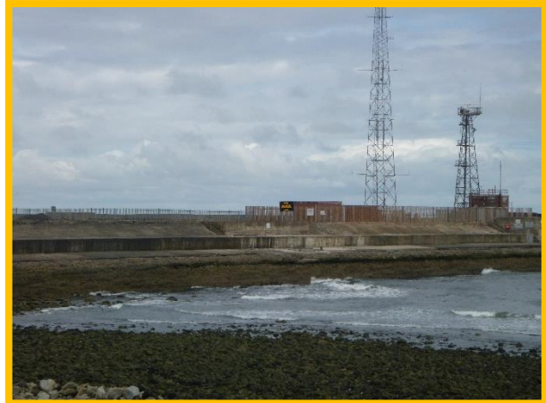
Potential voids visible beneath failed deck slab along eastern face (/C0506C01)
