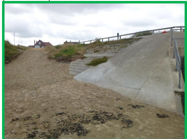
Transition of revetment into natural defence (/C0603C01)
