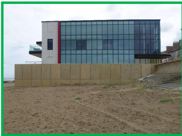
Cinema seawall in as-built condition (/C0602C05)
