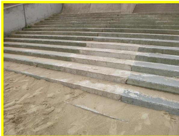
In situ concrete repair in fair condition (/C0602C04)
