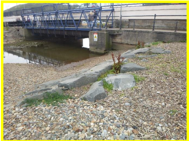
Grouted rock revetment to north of beck in fair condition (/C0704C06)
