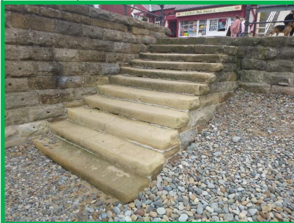
Beach access steps north of Saltburn Pier (/C0702C04)
