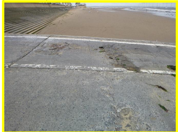
Slipway in fair condition with some spalling and abrasion damage (/C0602C02)
