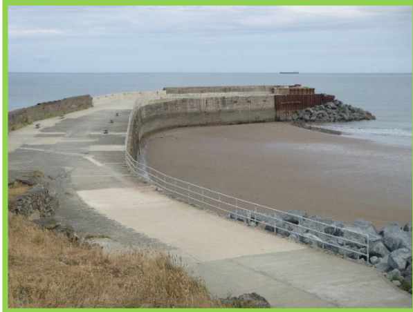
Inner face and deck of structure (Asset Ref No. 1221D901D0201C02)
