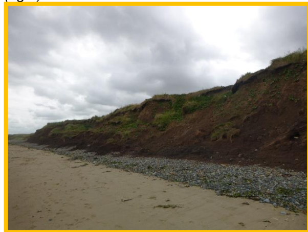
Looking south east along CBU E52/10 Partly Active in 2022.
