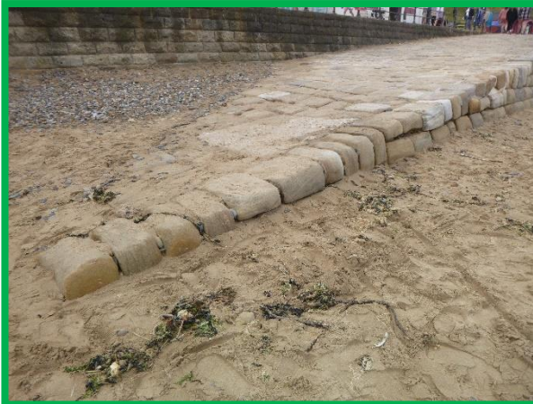
Repaired section of slipway coping (/C0702C04)
