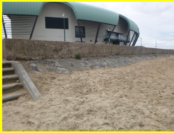
Grouted stone revetment, partially covered due to high beach levels(/C0601C01)
