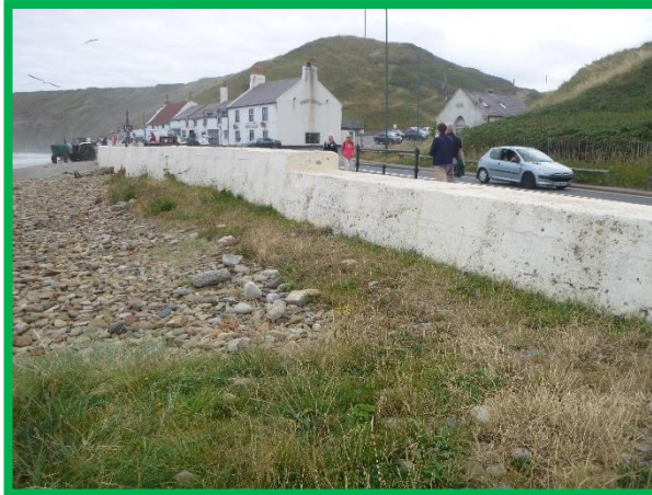
View looking west (/C0704C03)
